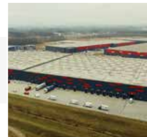
KOKOTÓW - Main Warehousez
